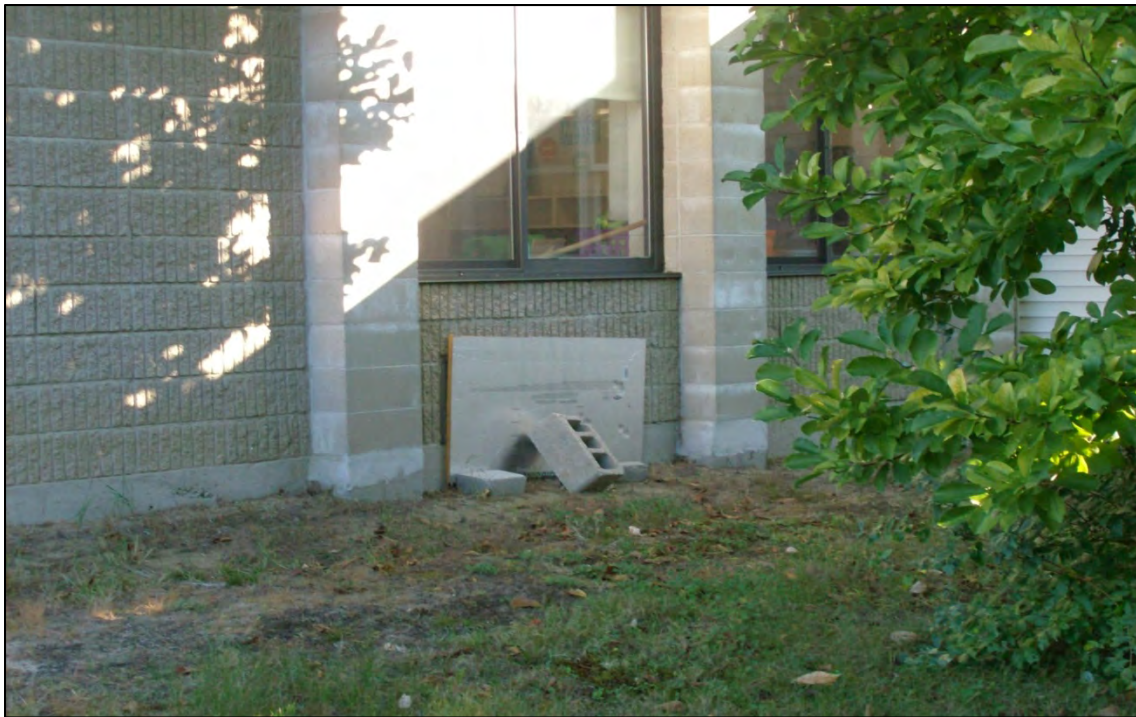
Unit ventilator grille blocked with foam panel.
