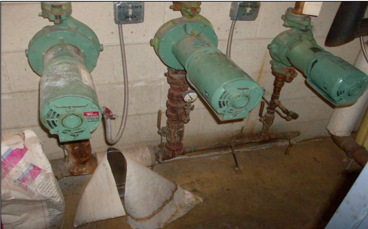
Hot water circulating pumps.
