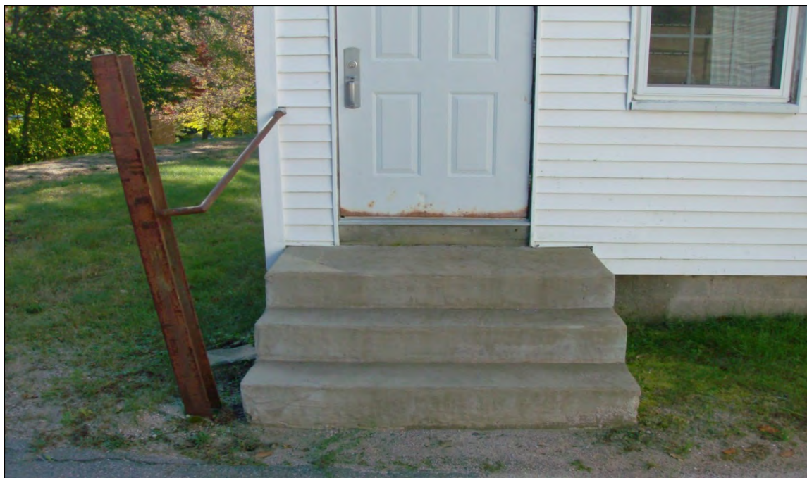
Door at Music Room. Door needs painting and railing should be replaced.
