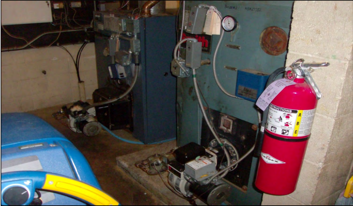
Two oil-fired boilers.
